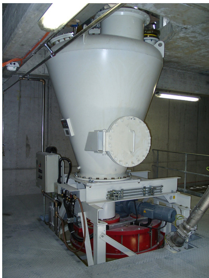
AF feeding with Pfister® TRW-D to the main burner
