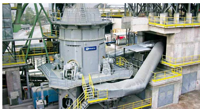
OK™ mill installation
