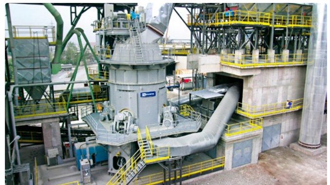
OK™ mill installation
