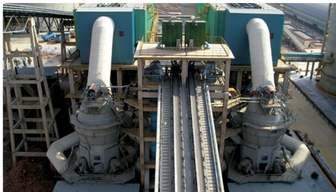
Twin mill installation
