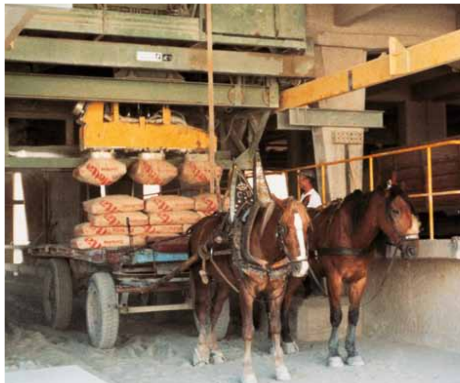
One of the first truck loader (Year 1969)
